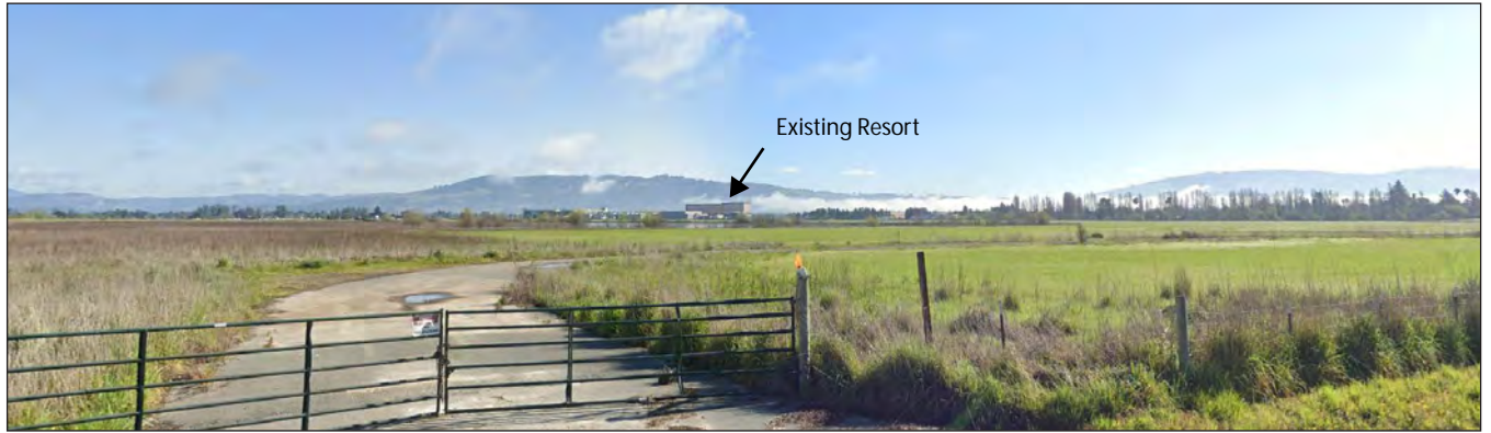
VIEW 1: Northeast View from Rohnert Park Expressway
